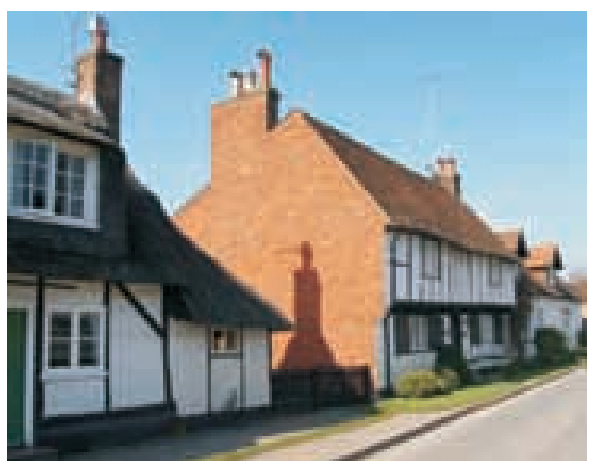
Jettied timber-framing, Stocks Road
