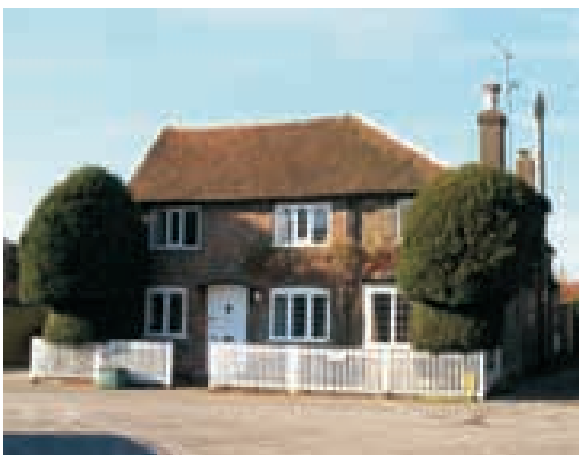
Old Post Cottage, Stocks Road
