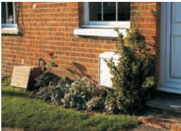
Meter boxes should be handled sensitively: exposed plastic boxes can be concealed in more appropriate timber enclosures
