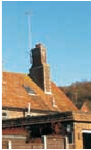
Rooflights visibly interfere with roofscapes
