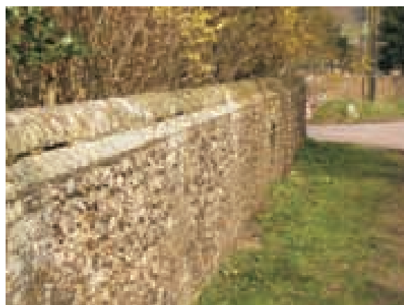
Wall to Church Farm
