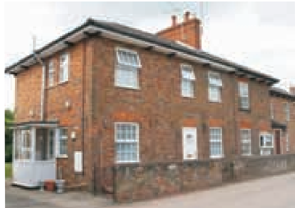
Introduction of plastic windows and doors, Trooper Road
