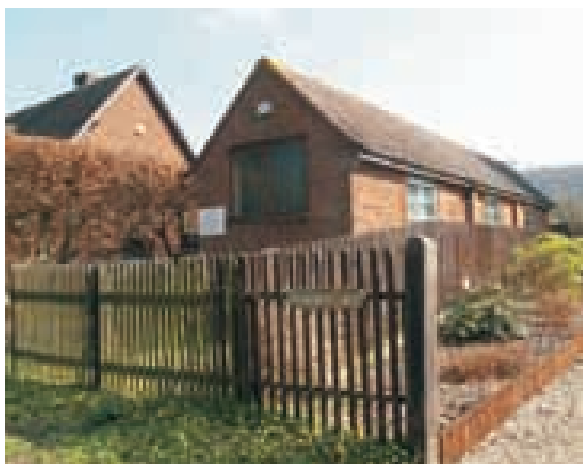
Telephone Exchange, Station Road
