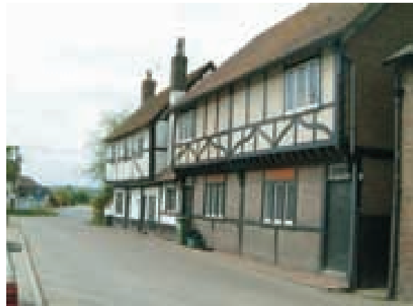
The house in the foreground replaced a barn to the former jettied house beyond, Trooper Road
